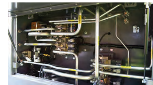
Steel pipework for better heat dissipation
